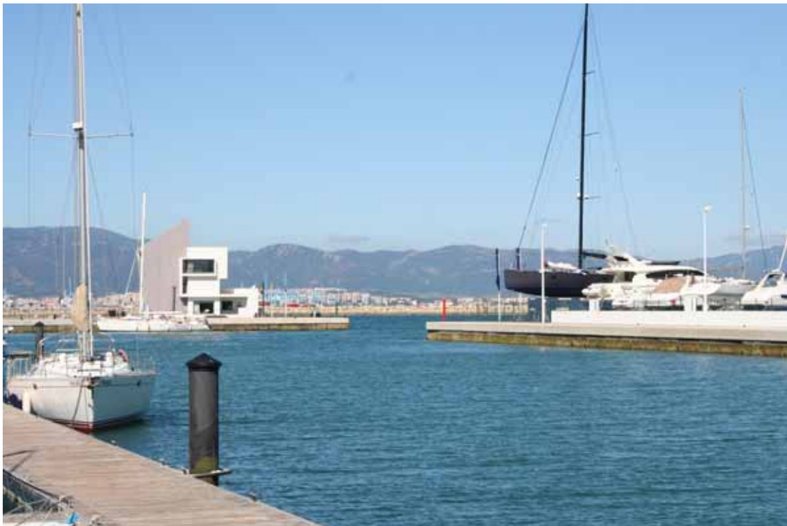
Marina Alcaidesa arrivals pontoon. Arrive where yacht (in the background) is moored, in front of office not at diesel pontoon which you will see first.
