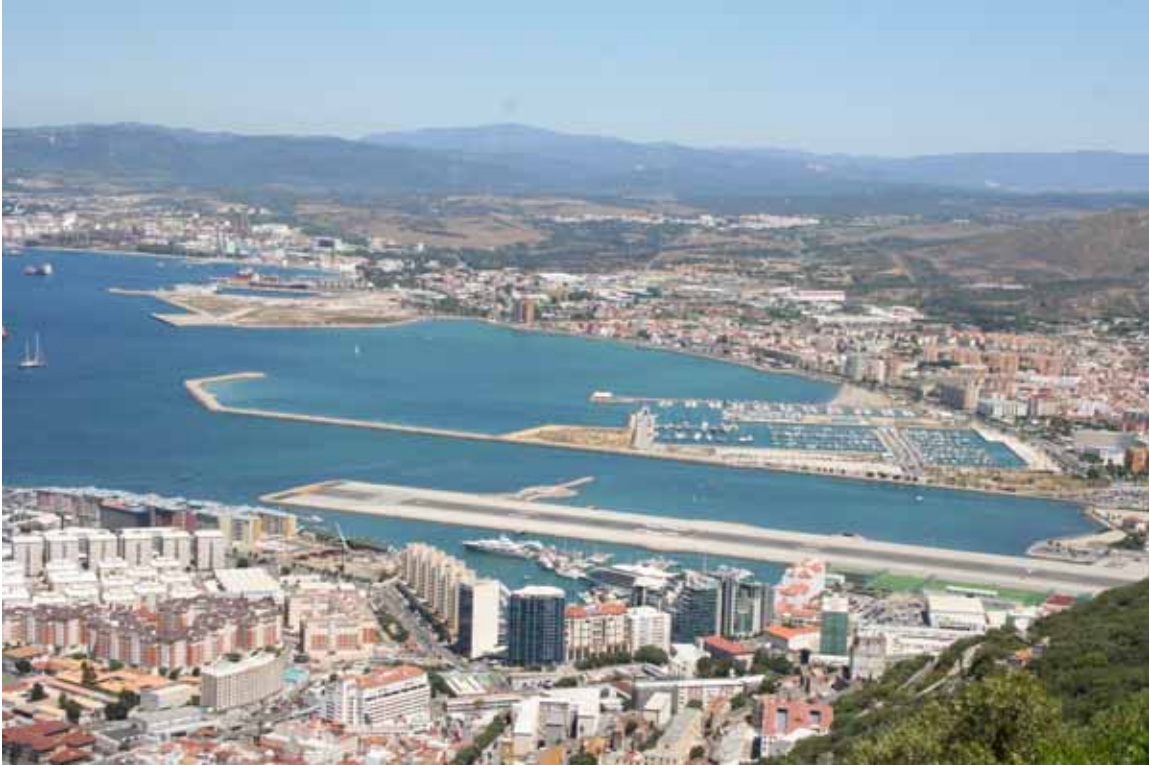
Essentially the main facilities in the area around Gibraltar. Marina Bay, Gibraltar (foreground) and Marina Alcaidesa, La Linea (central).
